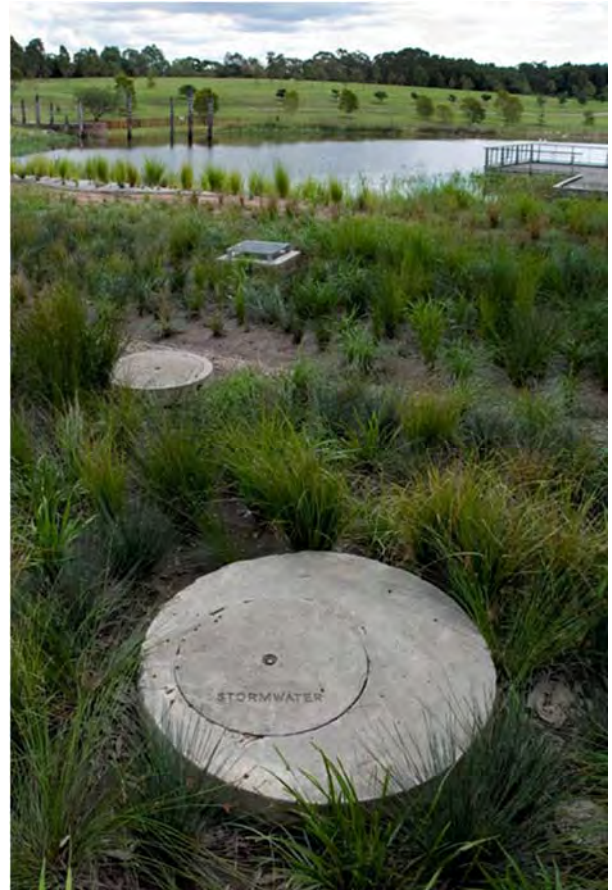
Sydney Park wetlands - stormwater
